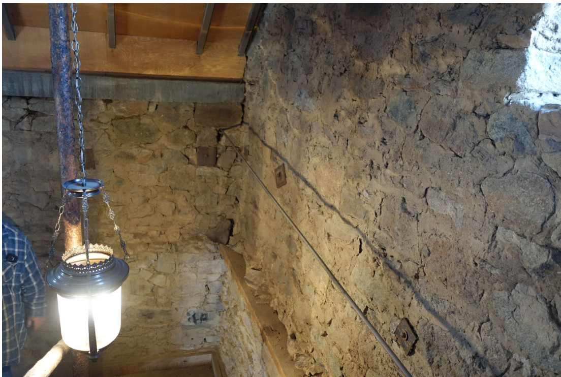
Stone Building – Game Room - FCA Building #4084 Description: View of the Limited Seismic Bracing.
